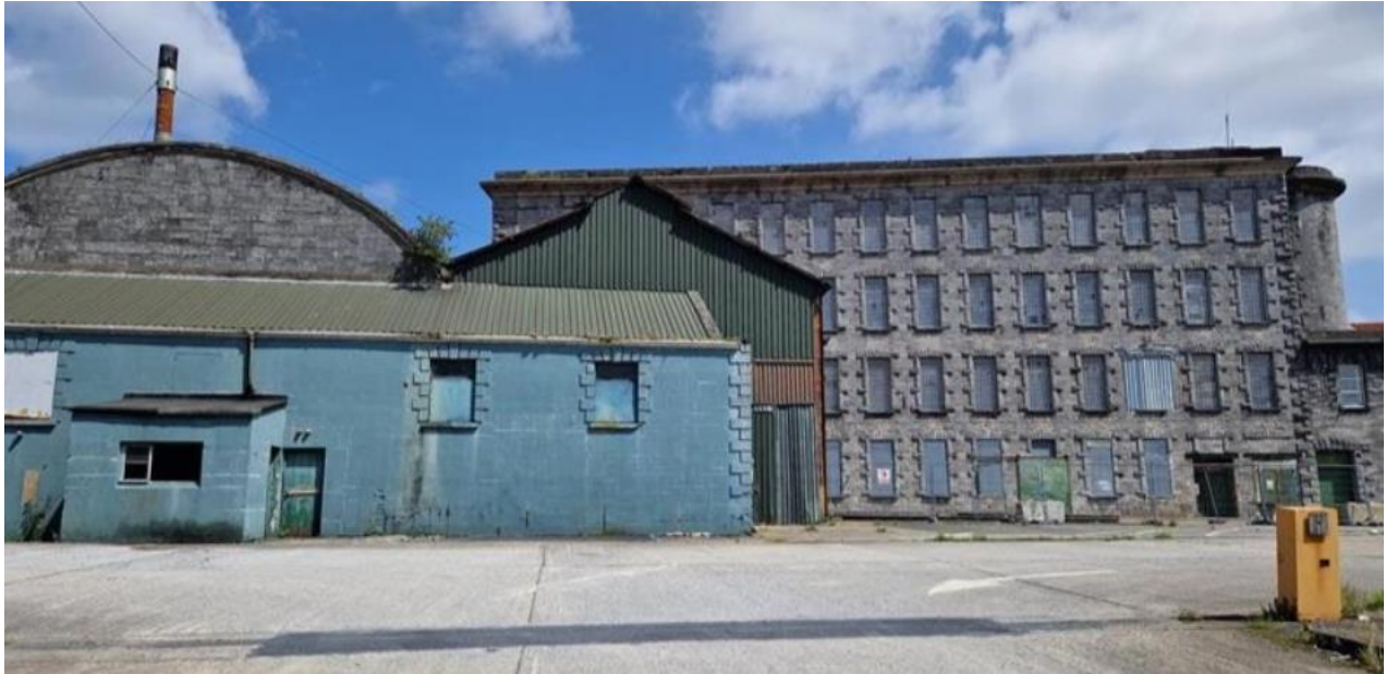
Figure 3-3 - View of Flaxmill area from North Circular Road
