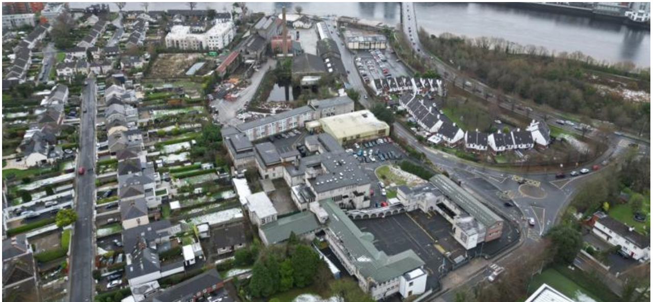
Figure 3-2 - Aerial view of site from the West
