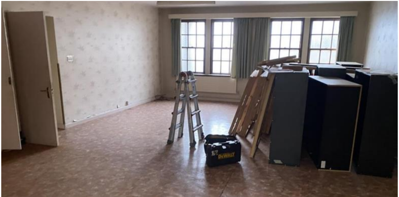
Figure 3-11 – Dining area within the Salesian School/Convent building (photo taken from Phoenix ACM Survey report)
