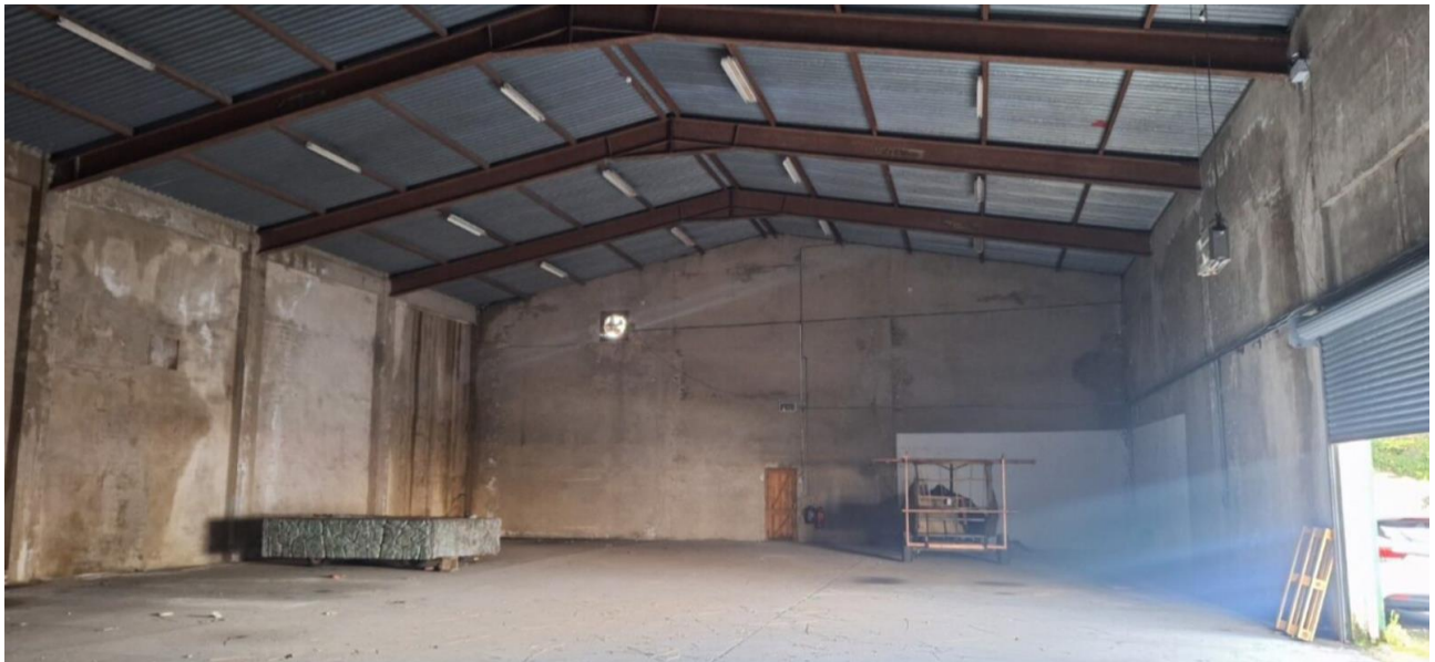
Figure 3-15 – Shipyard Warehouse – Internals.
