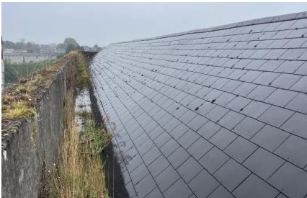
Figure 3-7 Concrete parapet and cement tile roof on the Flaxmill building (photo taken from Phoenix ACM Survey report)
