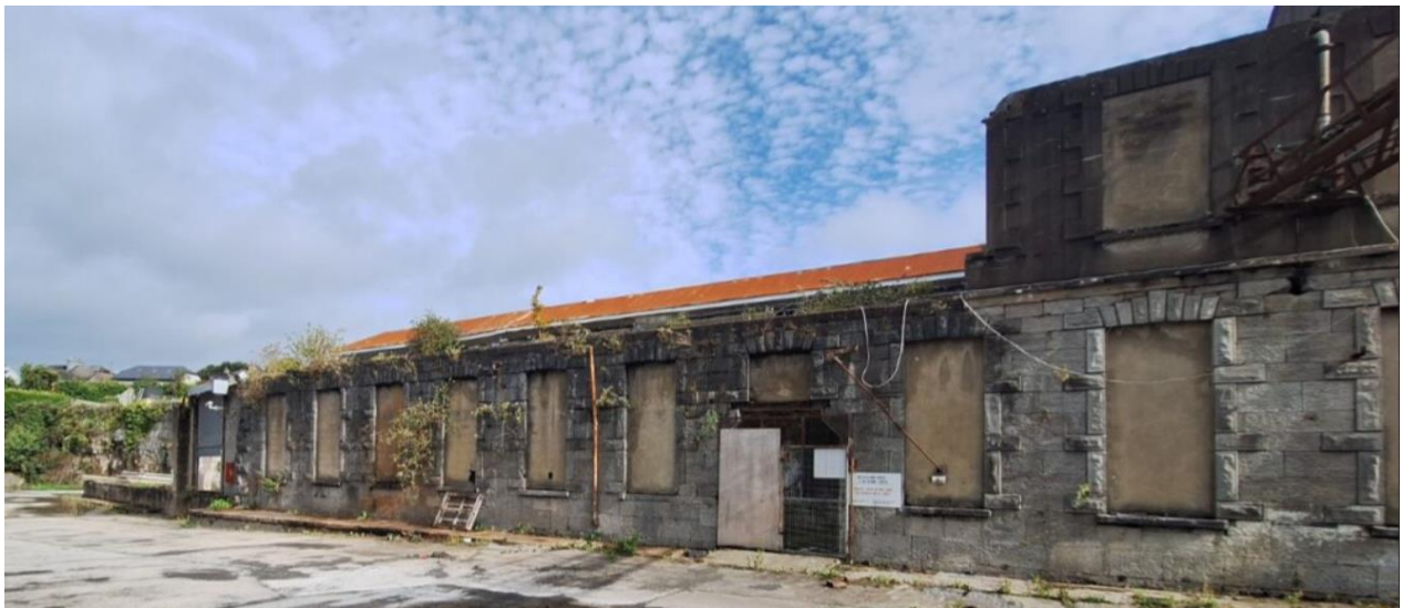
Figure 3-22 – Weaving Mill Lean Rear Lean-to
