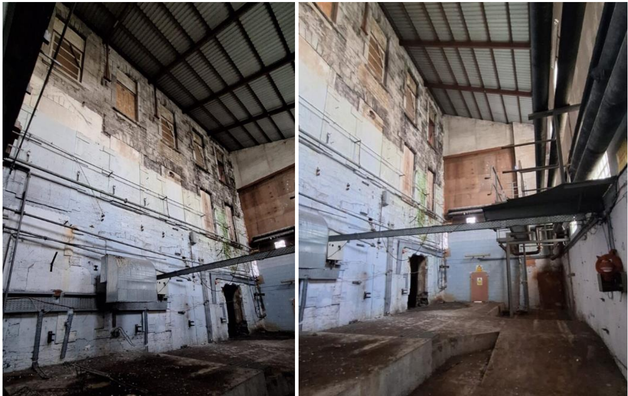
Figure 3-5 - View of Flaxmill extension internals (Lean to).
