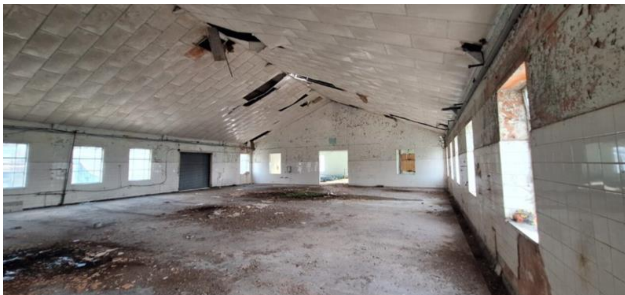
Figure 3-17 – Packaging Store and Offices – Internals.
