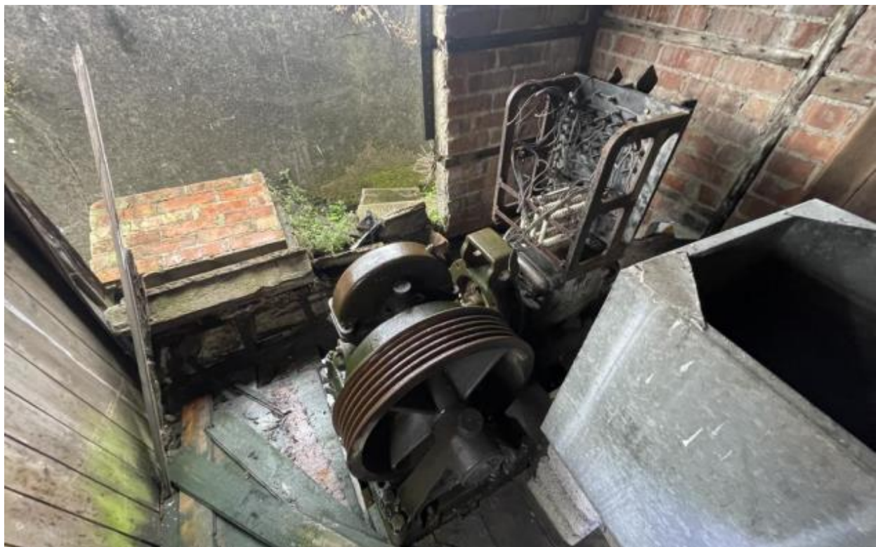
Figure 3-6 – Lift motor unit in the Flaxmill building (photo taken from Phoenix ACM Survey report)
